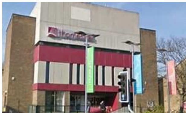
View of Thameside Complex from Orsett Road, Grays
